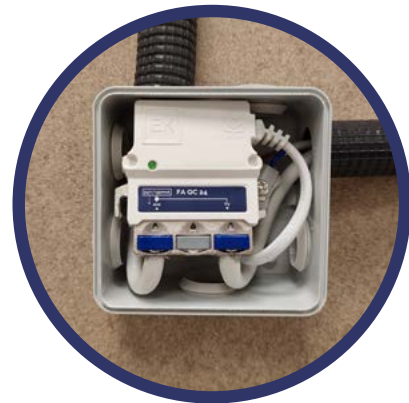
80x 80 mm junction box installation without F connectors
